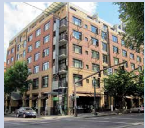
St Francis Apartments
